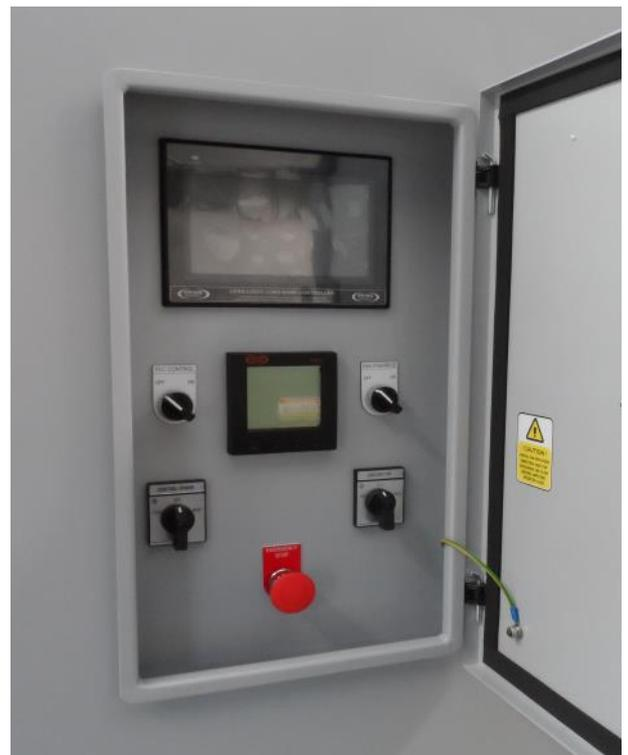
Control panel with 7" HMI and digital power meter
